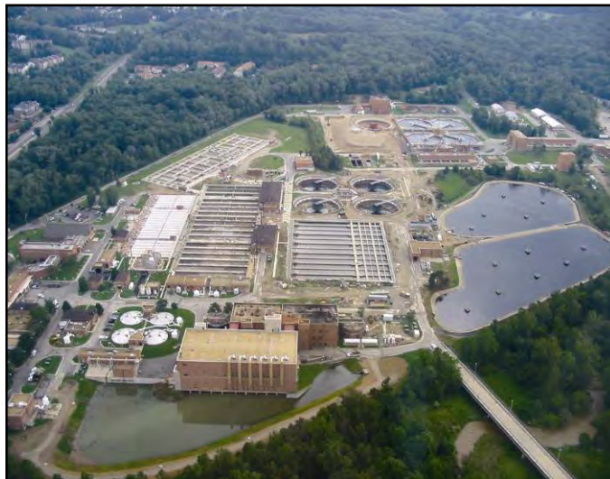
The County's wastewater treatment plant serves an estimated 364,500 households with public sewer service.
