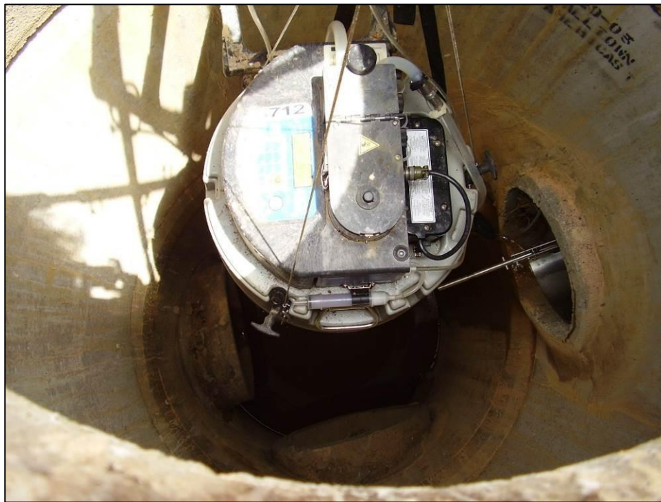
Automated sampler placed in manhole using hanger and spring ring
