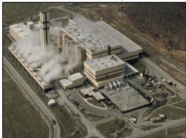
I-95 Energy/Resource Recovery Facility
