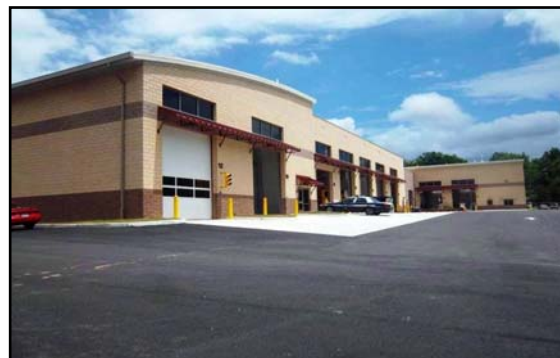
Renovation and expansion at the Newington DVS Facility in Mount Vernon District
