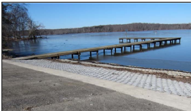
Replacement of Boat Ramp at Pohick Bay Regional Park
