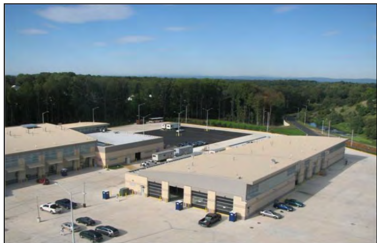
The West Ox Bus Operations Center commenced operations on June 29, 2009.
