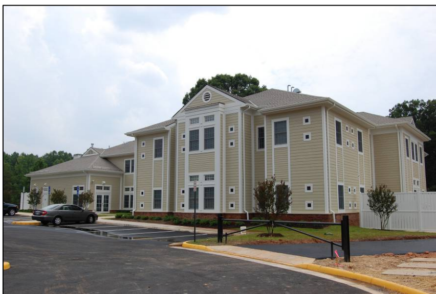
The new Katherine K. Hanley Family Shelter in western Fairfax County accommodates up to 20 families at a time.
